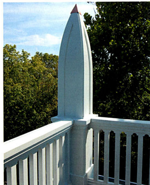
Like the originals, the new spires, which are made of Versatex PVC, are topped by copper. Photo: David Baio Photography
